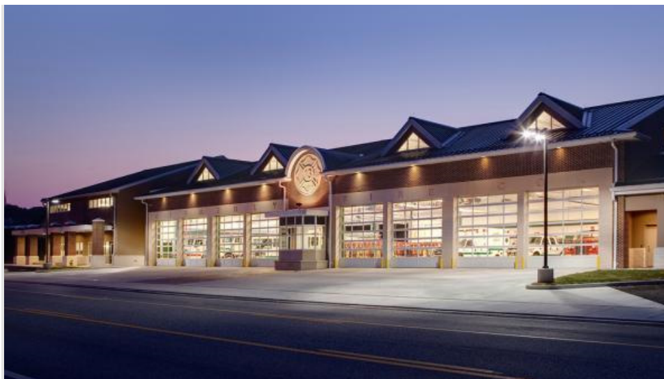
In the photo, the metal structure that houses the Singerly Fire Company in Elkton, Md.
