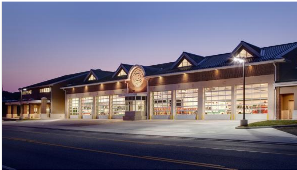
In the photo, the metal structure that houses the Singerly Fire Company in Elkton, Md.
