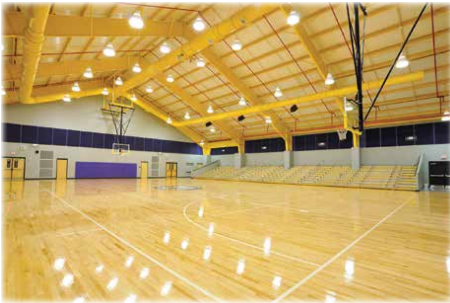
A metal building structural system provided the perfect column-free clear spans in the dining hall and gymnasium at the Louis and Josephine Buondonno Forum at St. Augustine Preparatory School in Richland, New Jersey.
