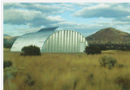
Introduced in 1941 for the U.S. Navy, a Quonset hut is a lightweight, prefabricated structure of corrugated galvanized steel. The name derives from Quonset Point, RI, where these were first manufactured. (Photo: Prometheussolar.com .)
