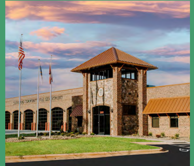
Cleveland Community VFD • Cleveland, N.C.
