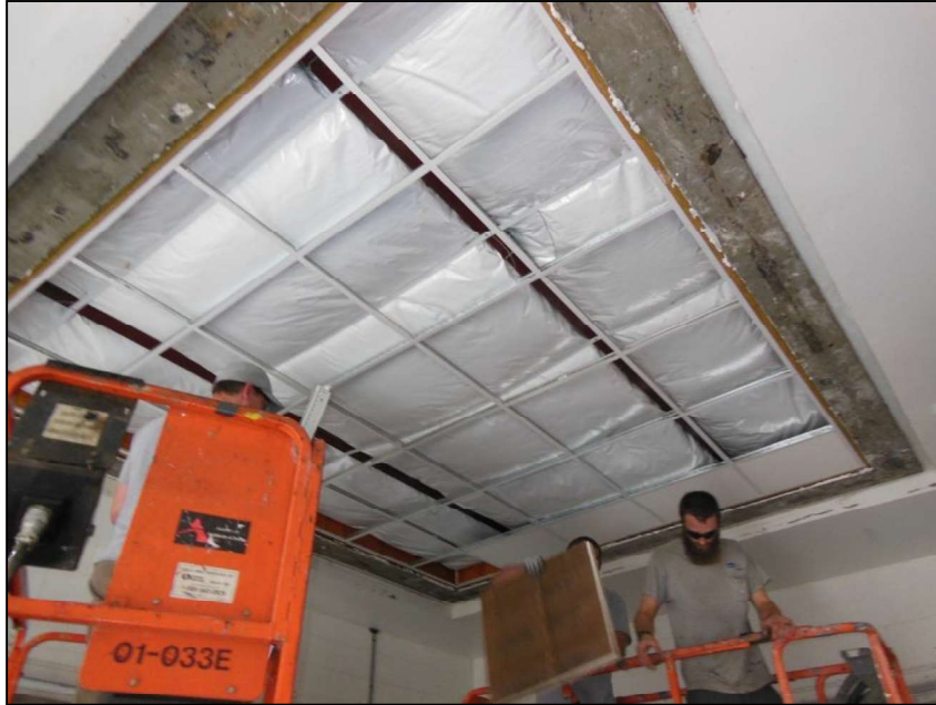
Construction of Test Specimen
