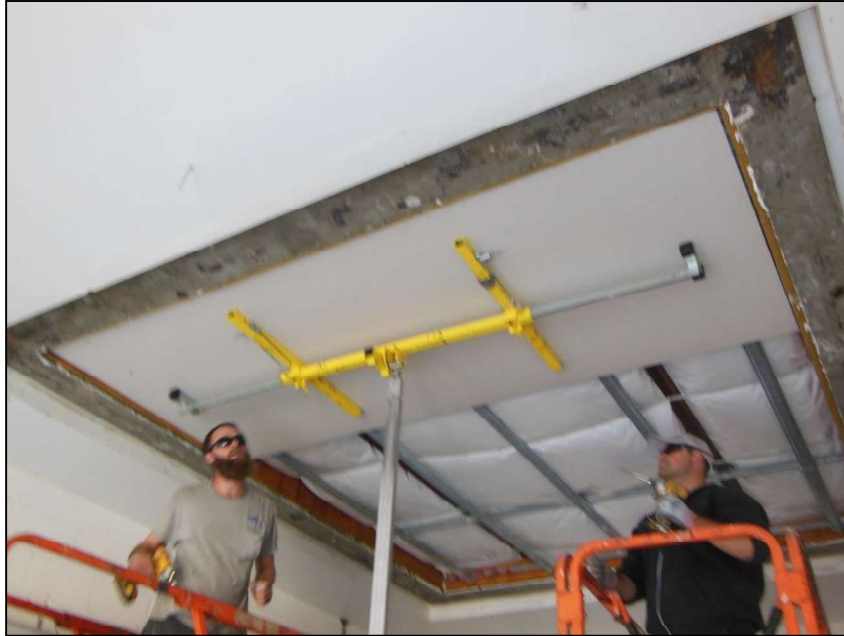
Construction of Test Specimen
