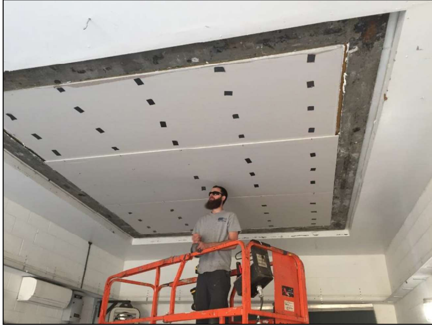
Construction of Test Specimen
