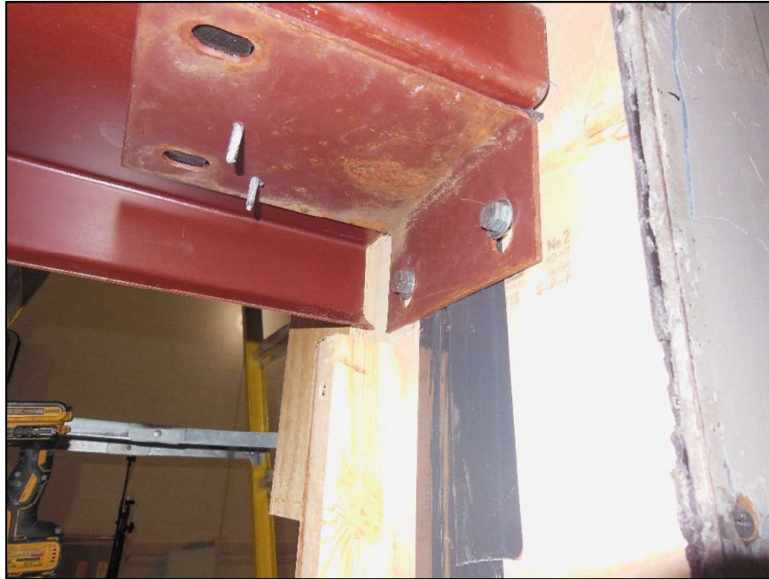
Girt with Support Bracket
