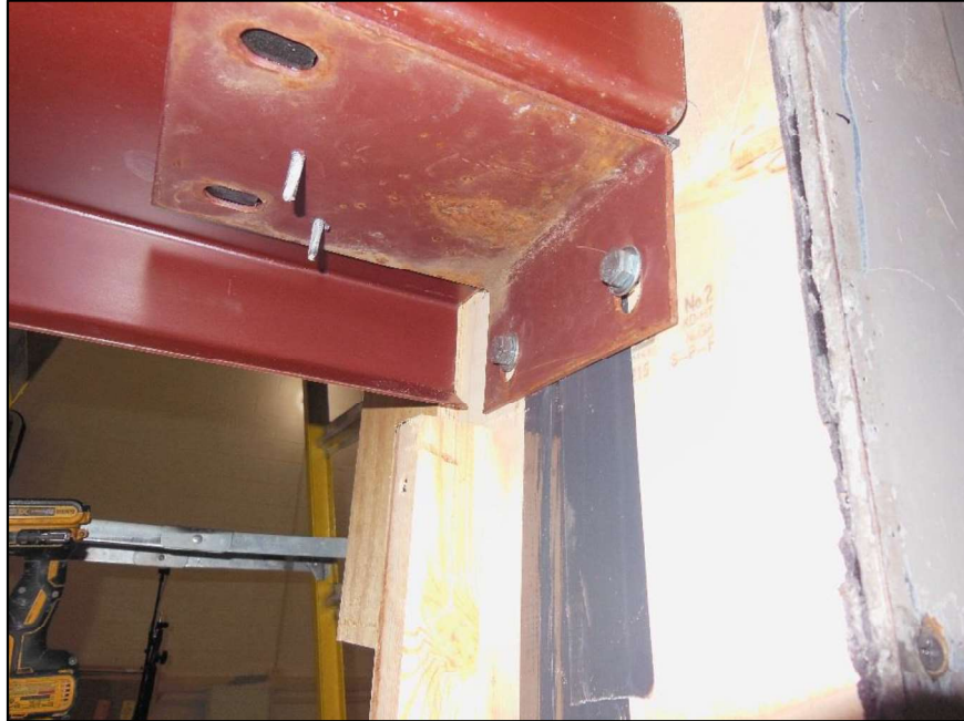
Girt with Support Bracket
