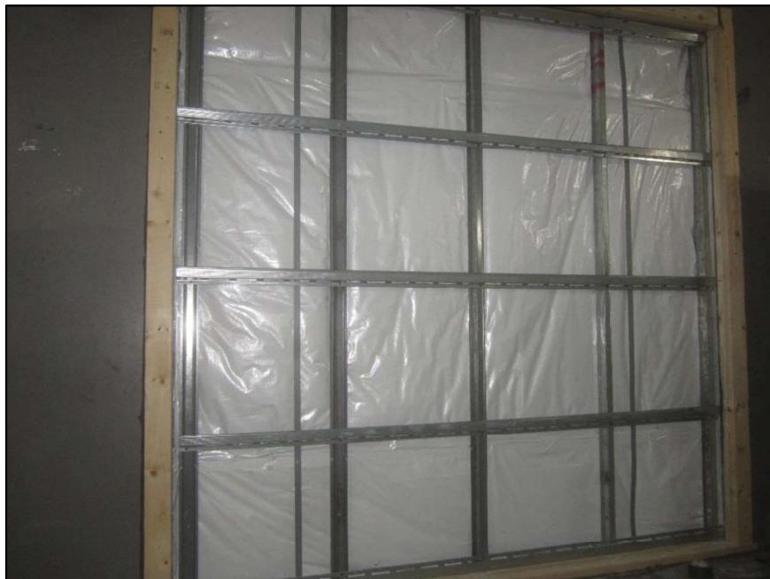
Hat Channel and Resilient Channel
