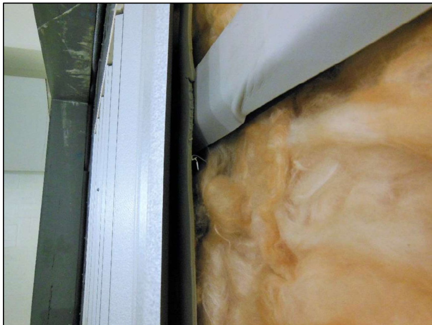
Isolator Foam with Metal Panel
