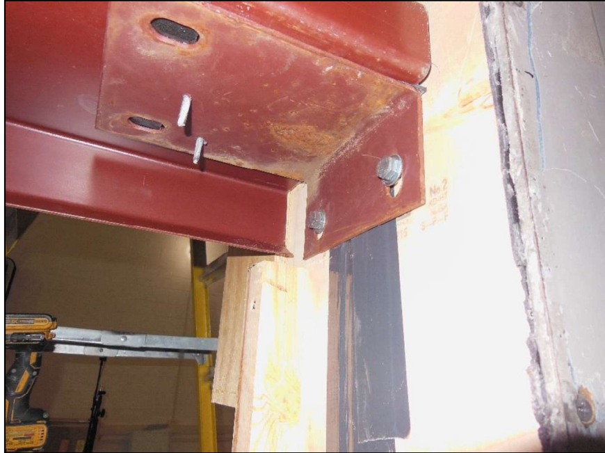
Girt with Support Bracket
