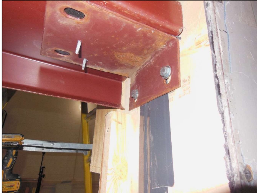
Girt with Support Bracket
