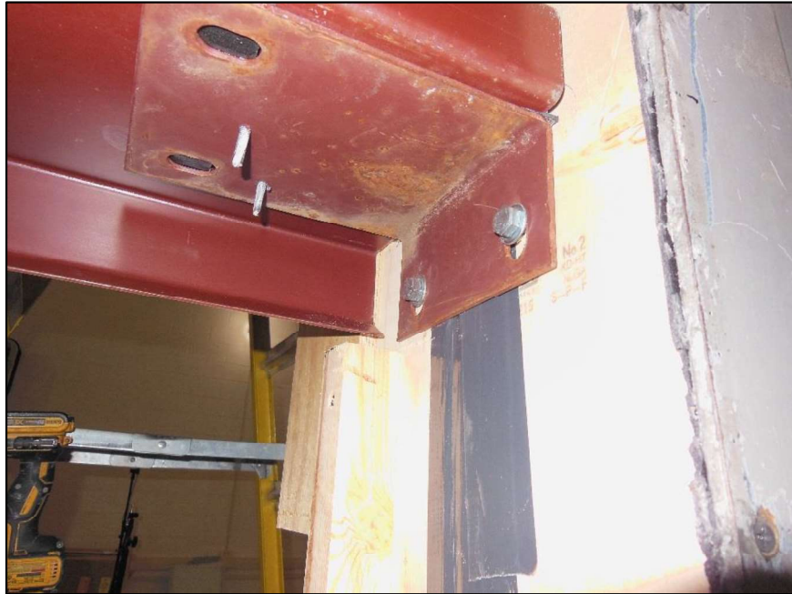
Girt with Support Bracket
