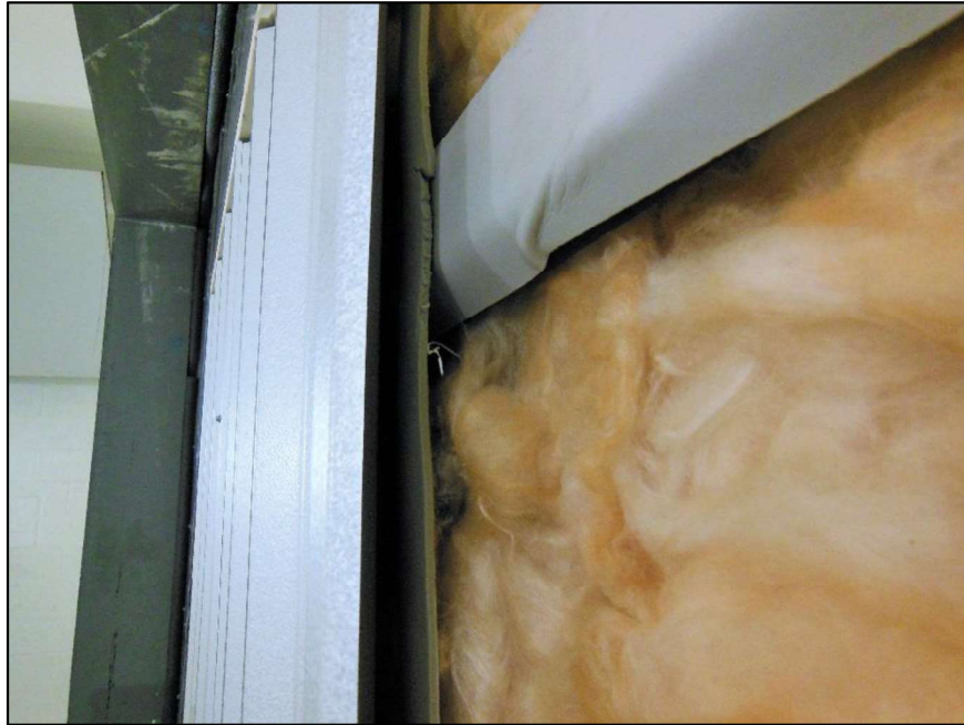
Isolator Foam with Metal Panel
