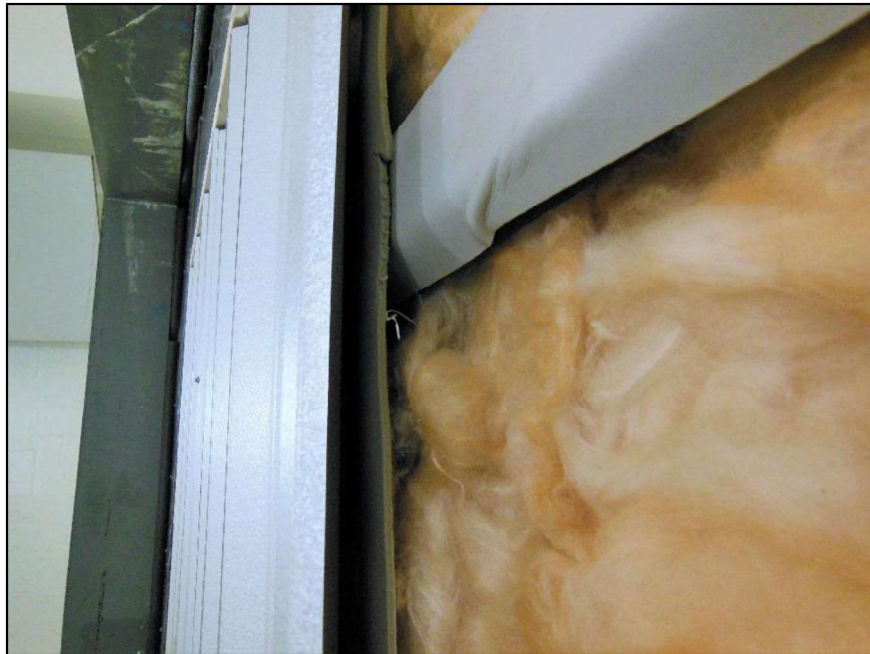
Isolator Foam with Metal Panel
