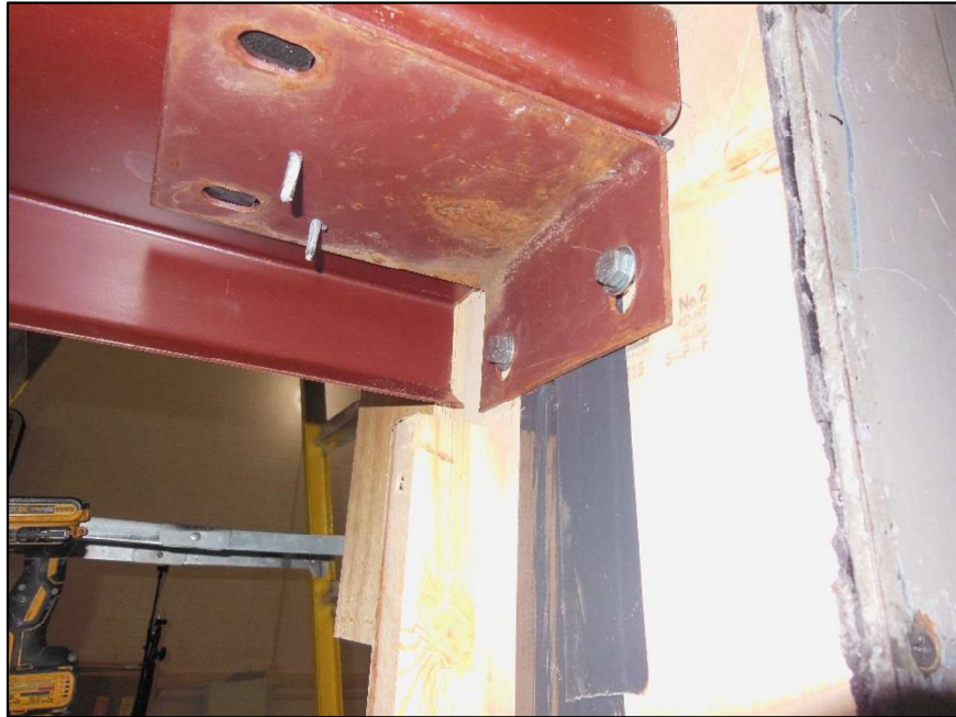
Girt with Support Bracket
