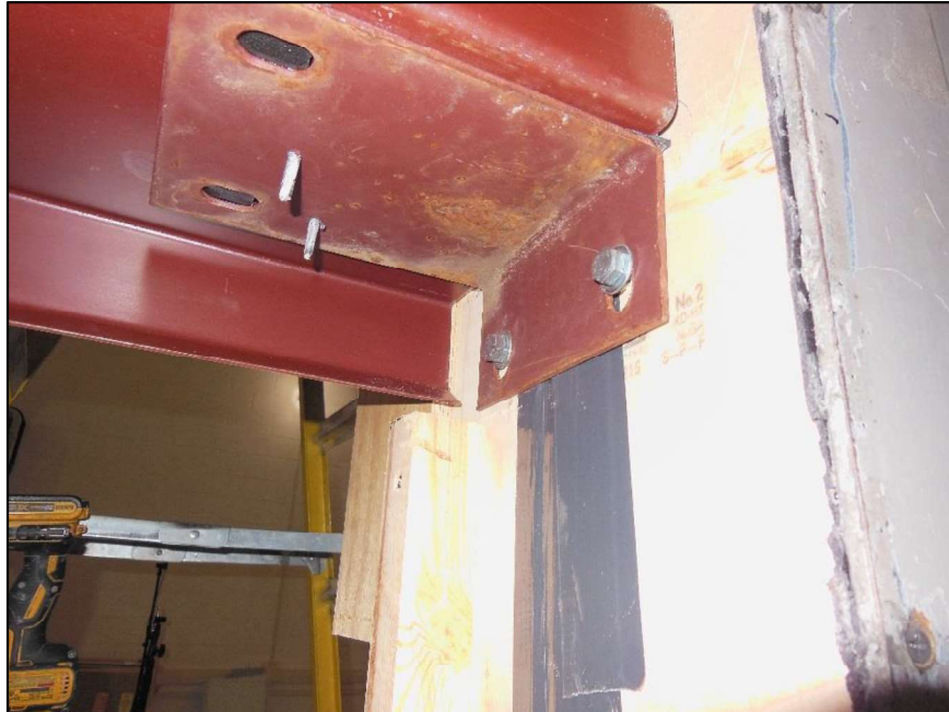
Girt with Support Bracket
