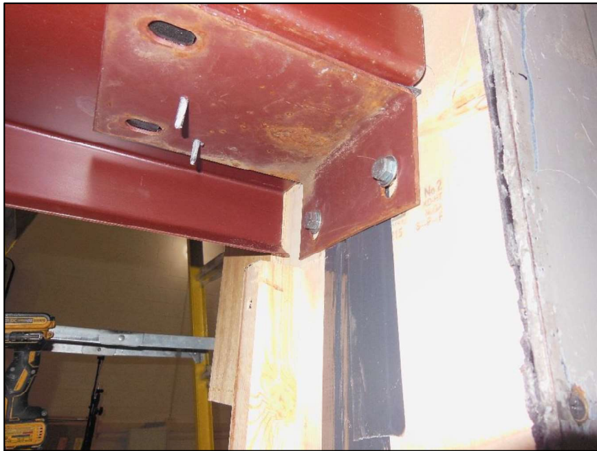
Girt with Support Bracket
