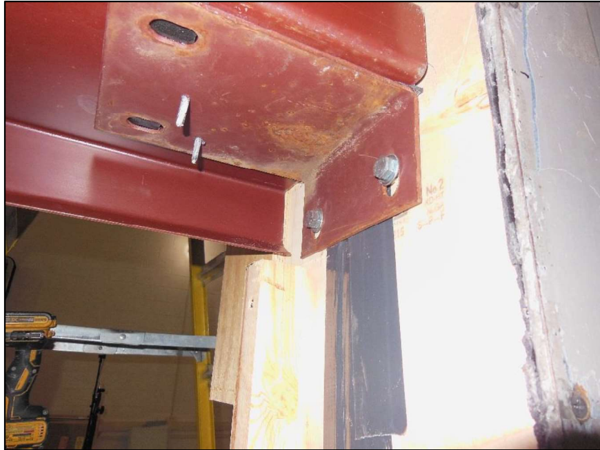
Girt with Support Bracket
