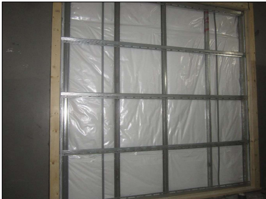
Hat Channel and Resilient Channel
