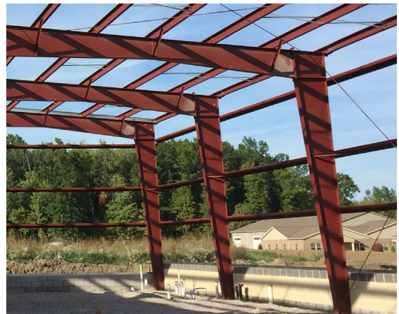
Girts and purlins attached to primary structural steel frames. Various types of bracing shown, such as x-bracing, flange bracing, girt/purlin bracing.
